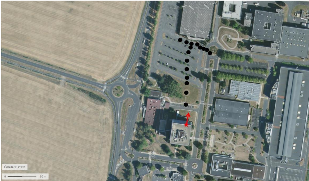
Figure 20: aerial view of the Nozay site and sector n°1 pointing towards a car park, the measurement points are shown in black. The antenna and its line of sight are shown in red.
